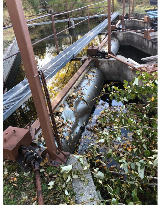
This screen was repaired after a tree fell and caused major damage.
